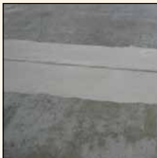
Slab Curl Removal
