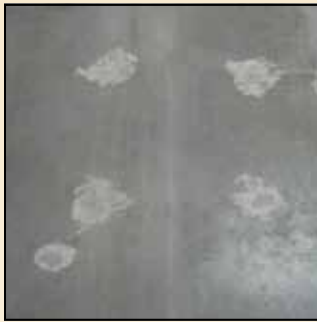
Bolt Hole Repair
