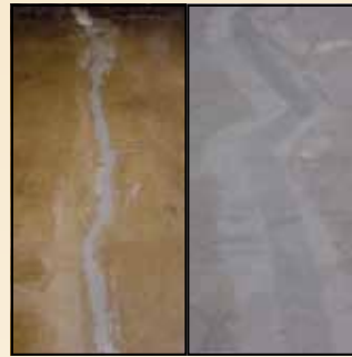
Crack Filling & Rebuilds
