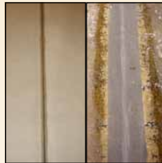
Joint Filling & Rebuilds
