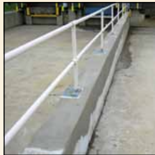
Exterior Concrete Repair
